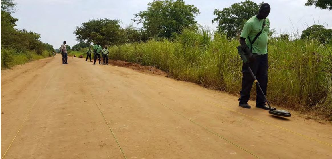
*The majority of the suspected mined roads in South Sudan are devoid of vegetation and believed to only be contaminated with anti-vehicle mines. As such clearance is done using a combination of dual sensor detectors and mine detection dogs in a deployment style that achieves 1km of road clearance per day (8,000m<sup>2</sup>/day). Therefore, road tasks are disaggregated from other demining tasks, as the speed of clearance is so different.*
