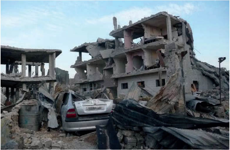
Massive destructions after fighting in a Syrian city © Handicap International/Philippe Houllat
